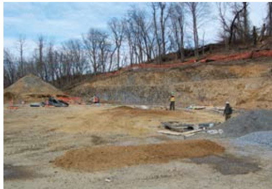
Workers prepare the ground for the new shelter.
