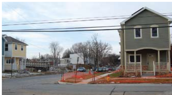
The intersection of Swatara and 16th is busy with residential construction, including a zero-net energy use home (far right).
