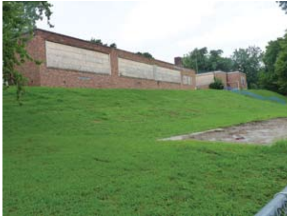
The site of the shuttered Thomas Morris Chester School in Riverside, which soon will be razed to make way for a new synagogue for the Chisuk Emuna congregation.
